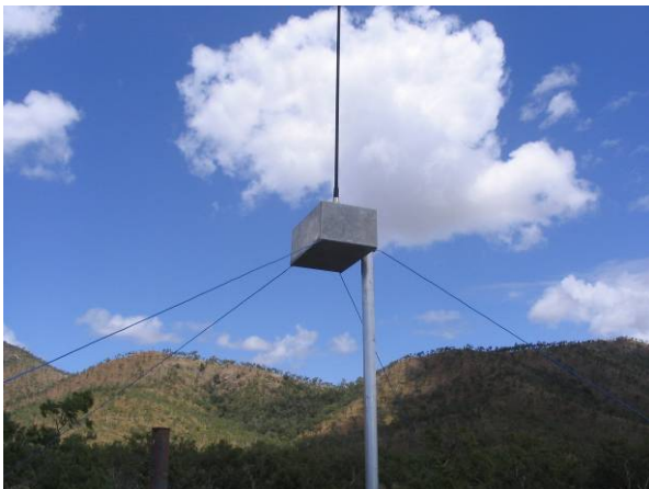
Figure 5. Node installed with radials
